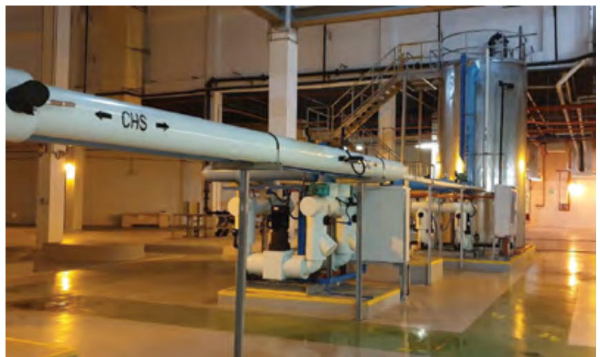
The Phase-Change Material thermal energy storage system installed at Keppel DHCS' Changi Business Park district cooling plant. Image: Keppel DHCS.
