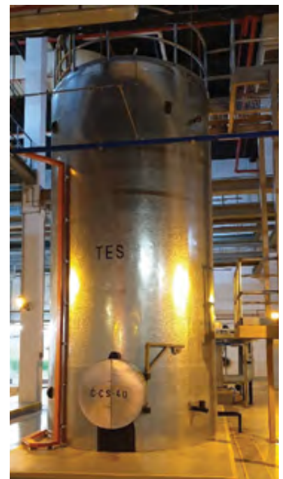
The Phase-Change Material thermal energy storage tank. Image: Keppel DHCS.
